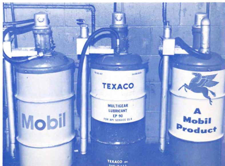
A closer view of the three Jet Power Lubrication Pumps that are delivering chassis grease, gear lubrication, and motor oil to the hose reel unit.
